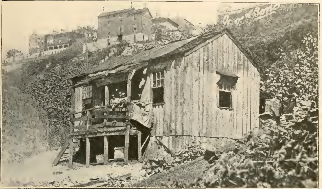
KERSEY COATES TERRACE, BEFORE GRADING.
